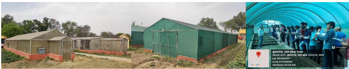
Glasshouse and Net house (Protected cultivation structure)
